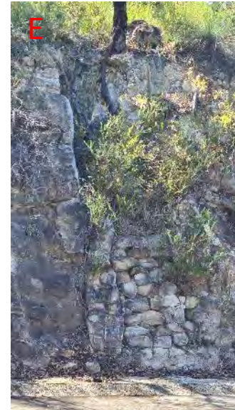
West Head Road Dyke
